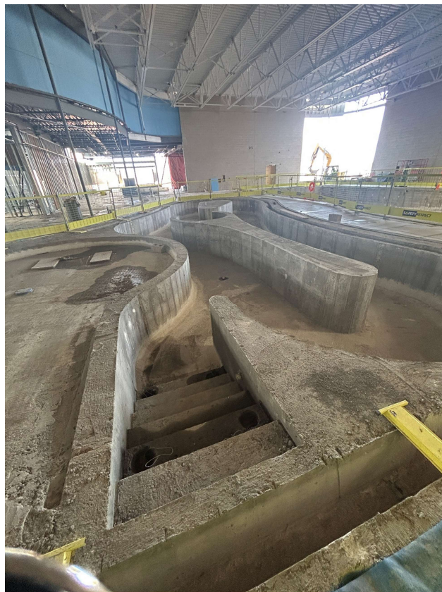
Figure 6. EdenCrete was used in the floor and walls of the pools
