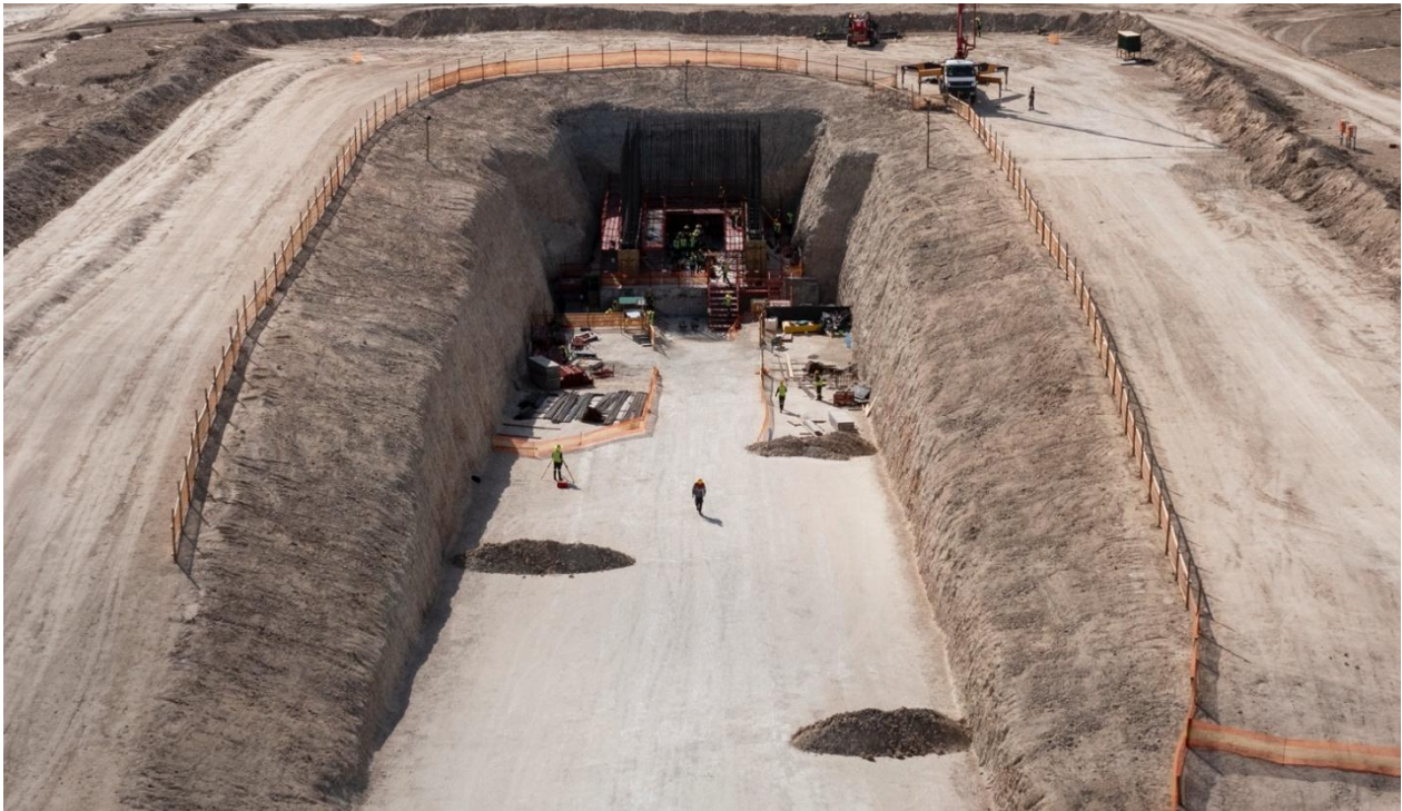
Figure 4: The first concrete pour at the primary crusher site has been completed. A total of 500m 3 was poured at an average flow rate of 40m 3 per hour.
