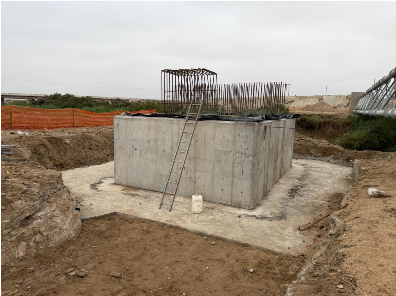
Figure 7: The permanent water supply pipeline bridge base to cross the Swakop River is nearing completion.
