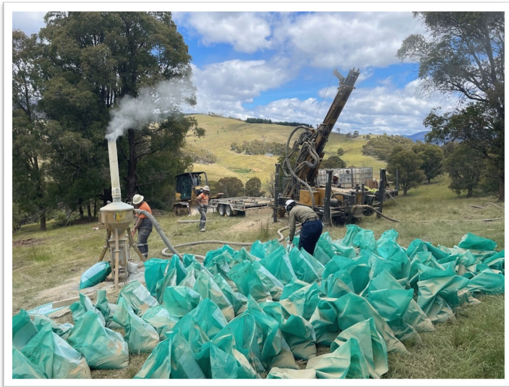
Figure 1: Reverse Circulation (RC) drilling on site at EL7073 Cobungra.
