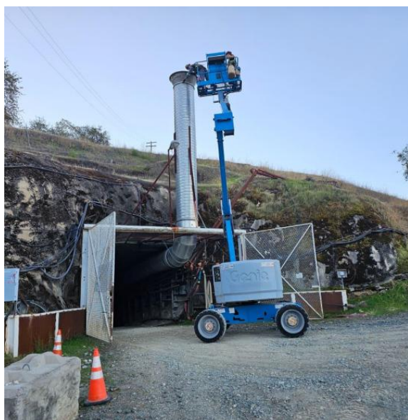
Figure 8: 4x4 articulated boom, checking ventilation tower 8 .
