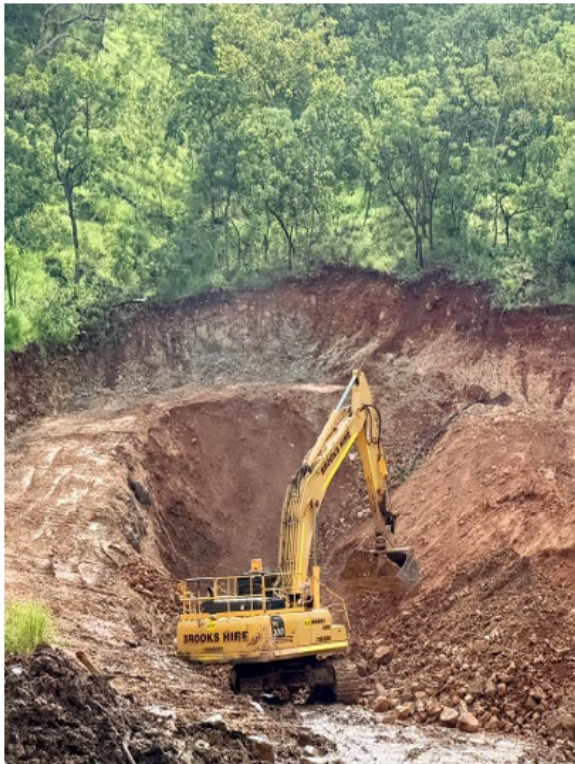
Plate 1 – Ground stability and box cut earth works
