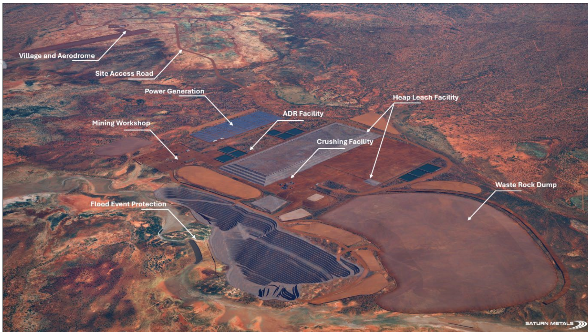
Figure 3 – Apollo Hill Open Pit Mine and Heap Leach Processing Gold Project – PFS Design Rendered Visualisation.
