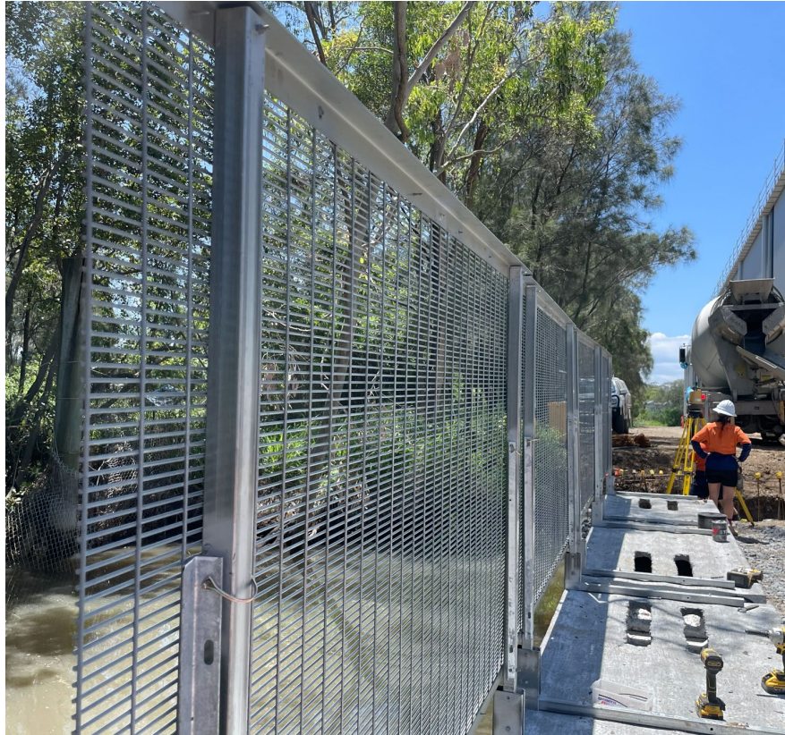
Image 1. Pre-installed PIEPS® edge safety system
