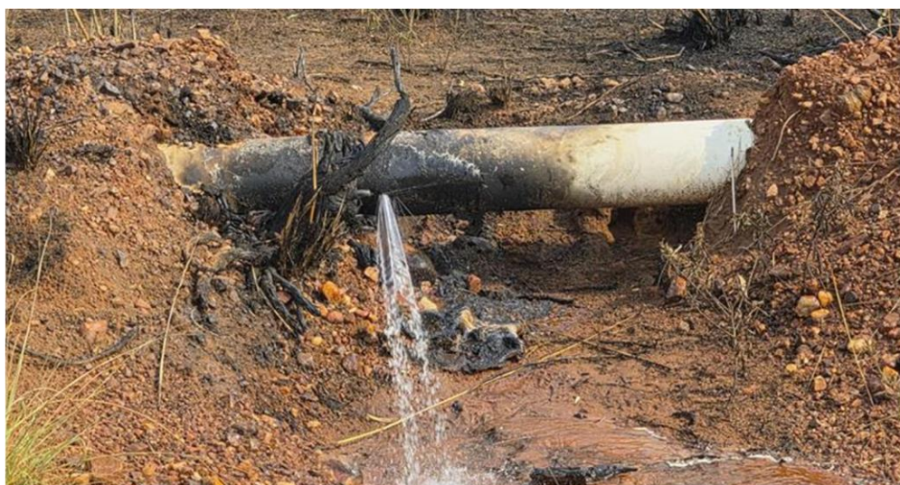
Figure 1: Water pipeline damage due to bushfire
