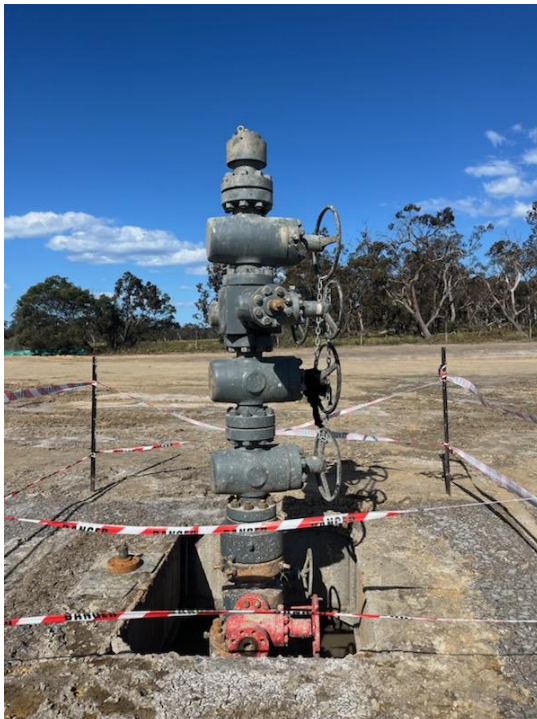
Figures 2 & 3: Wombat-5 production wellhead and cleared wellsite
