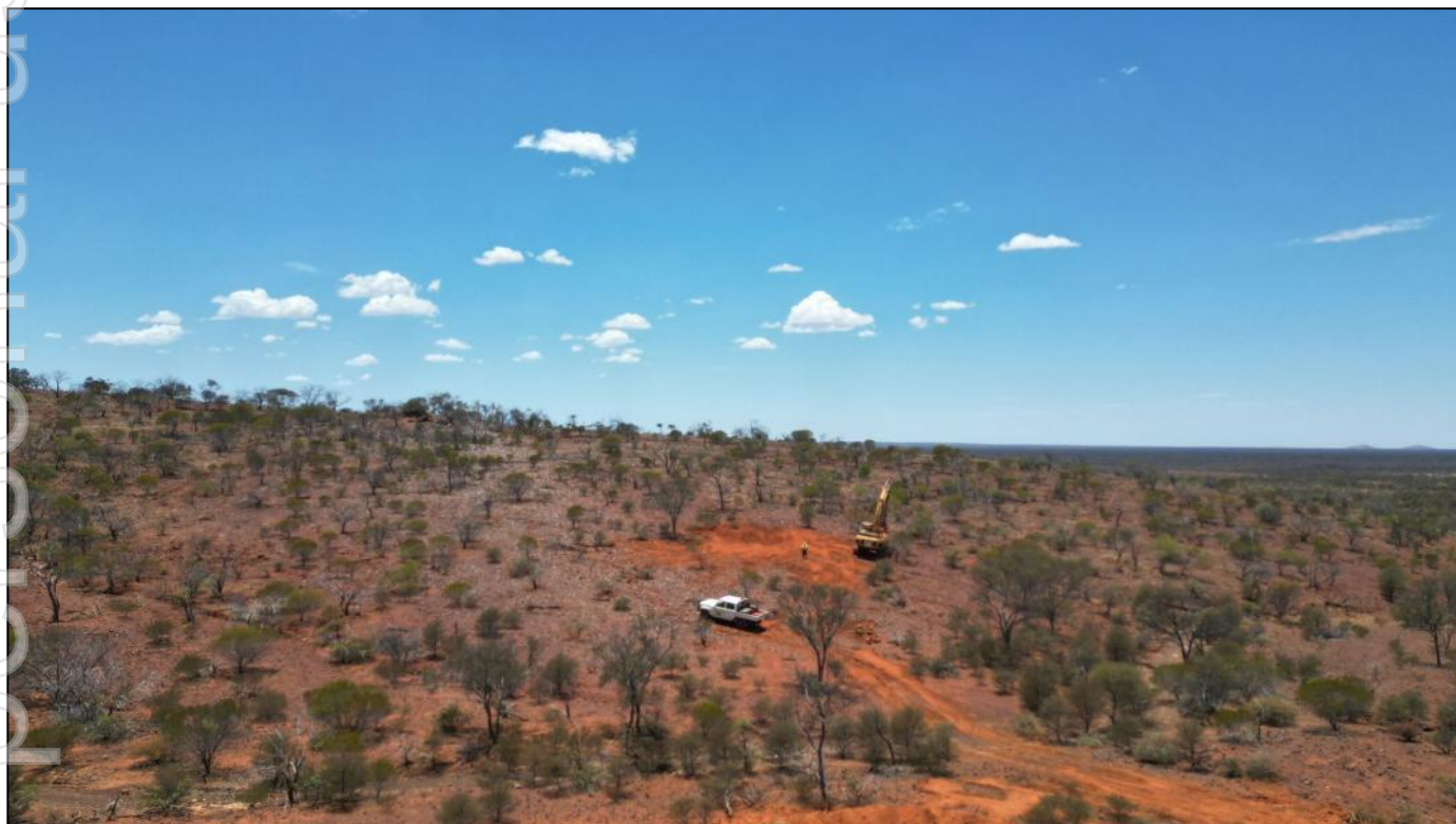
Figure 3: Drill pad preparation at Mt Kersey
