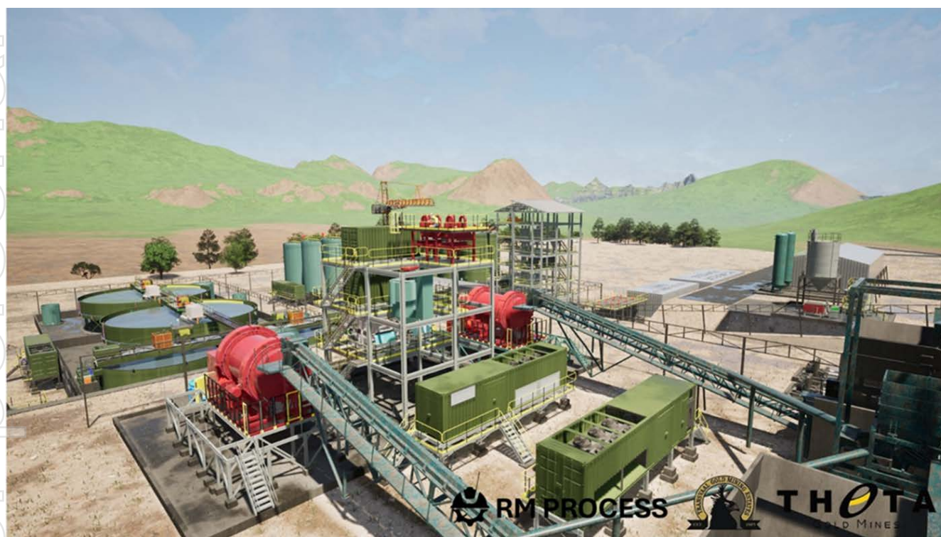
Figure 23: 3D rendering by RM Process of the Milling Circuit in Foreground
