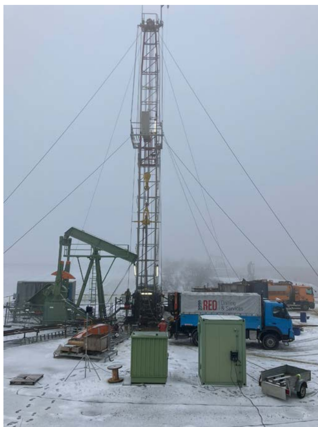
Figure 3: The RED Drilling & Services AW102 rig conducting workover operations on a Vienna Basin Field oil well
