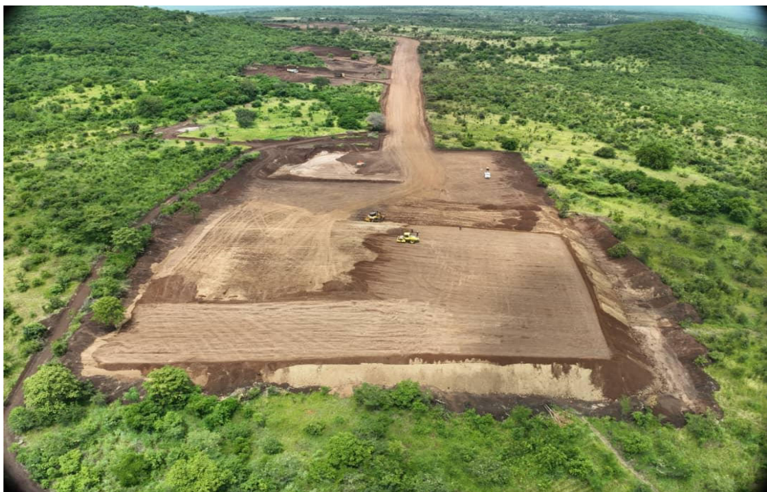
Figure 8: Explosives magazine precinct earthworks completed, with the platform and access alignment prepared to support safe storage and controlled supply for upcoming drill-and-blast operations.
