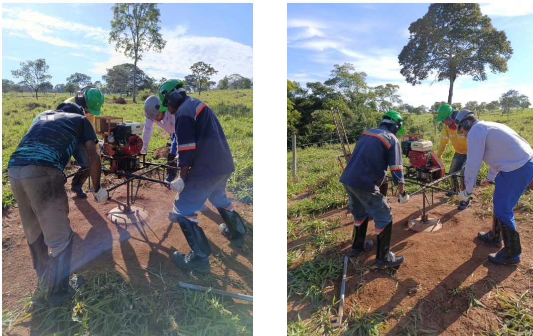
Figure 6 - Auger drill teams at the Piracanjuba prospect, 28 th January 2026.
