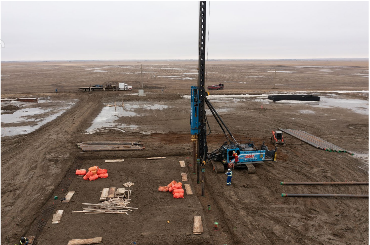
Figure 1: Installing piles for facility foundation at Pad #1
