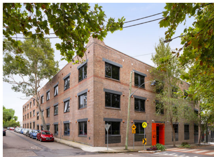
43-45 Australia Street, Camperdown, NSW
