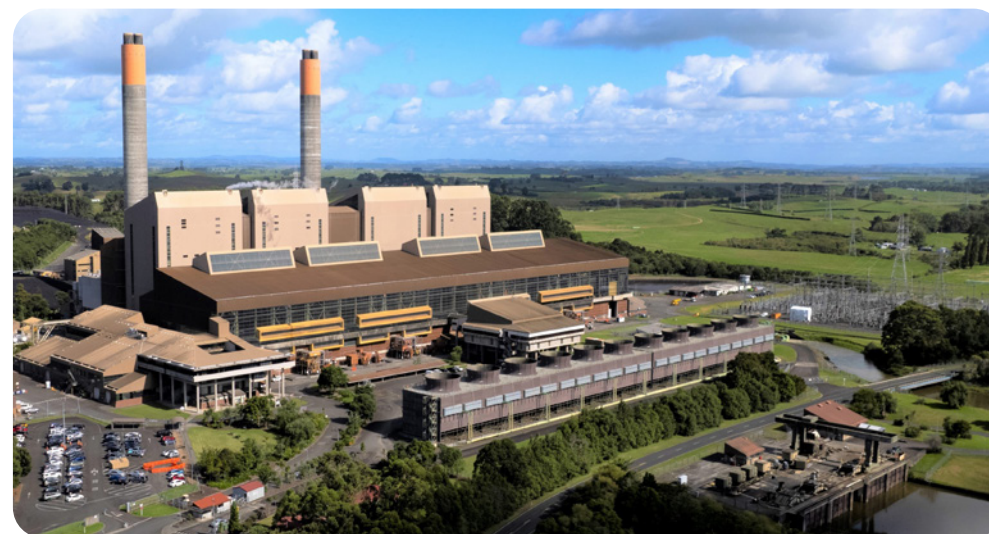
Huntly Power Station
