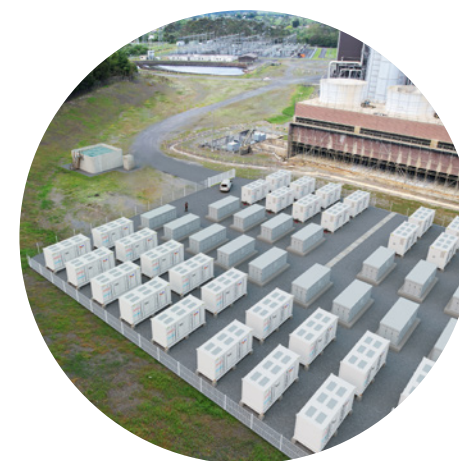
Artist's impression of the battery installation at Huntly Power Station.
