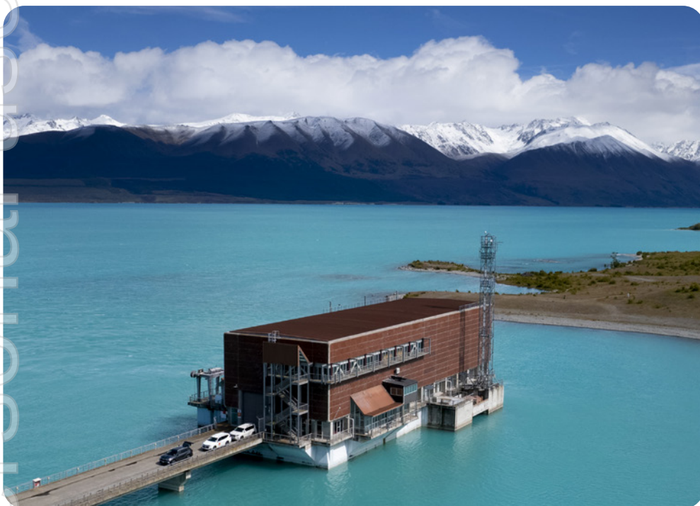
Tekapo B Power Station
