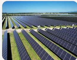
Lauriston Solar Farm
