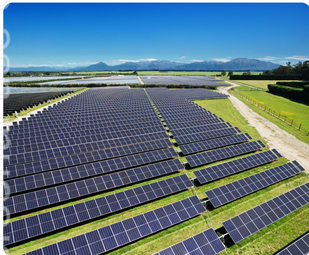
Lauriston Solar Farm
