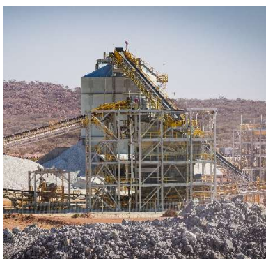
Commissioned paste plant
