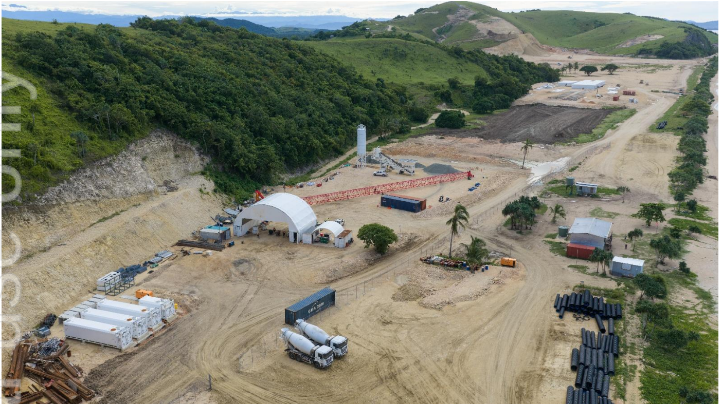
Photo: Construction progress at the Central Lime Project
