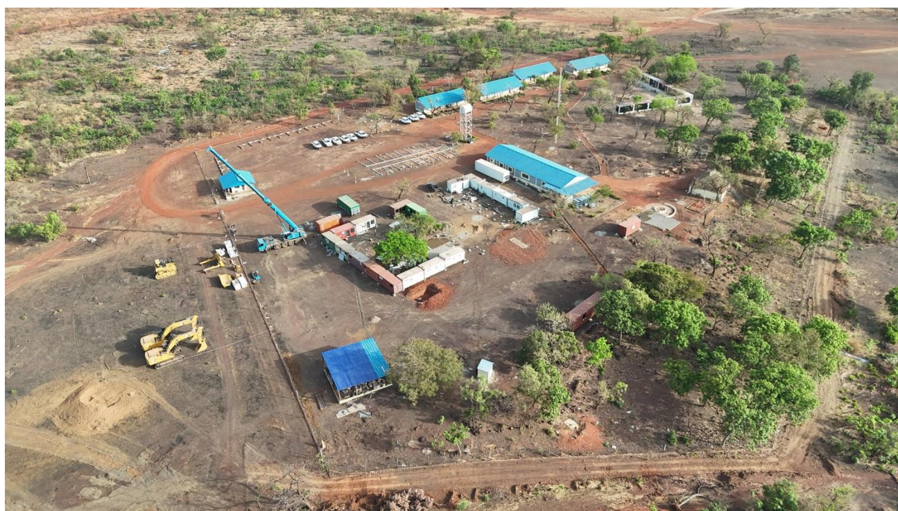
Photo 3: Construction of new accommodation facilities at the Kobada Camp
