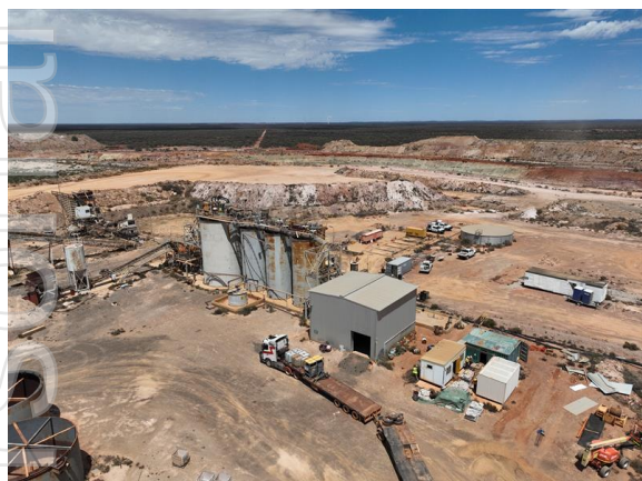
Clearing of old mill site completed (Dec'25)
