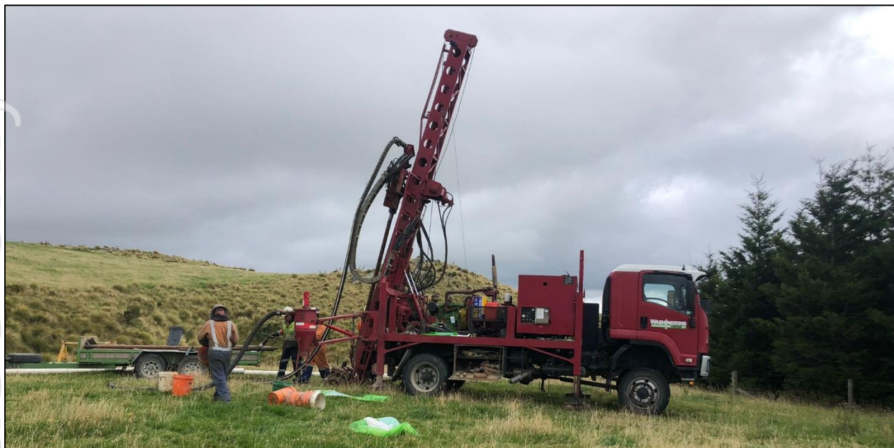
Figure 1 Drilling rig on site at Lammerlaw
