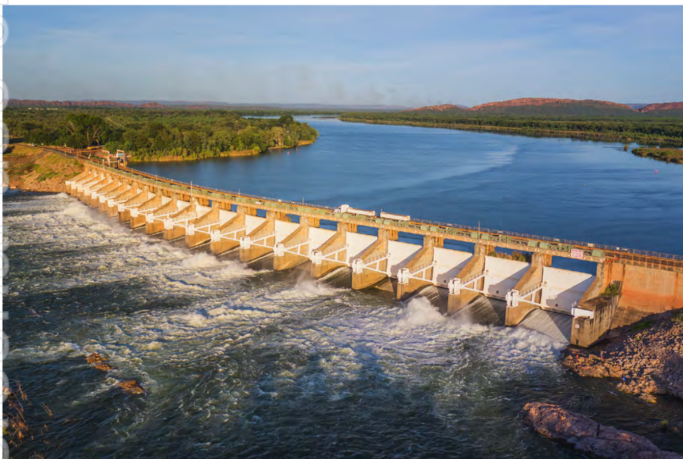
Figure 60: Diversion Dam, Kununurra.
