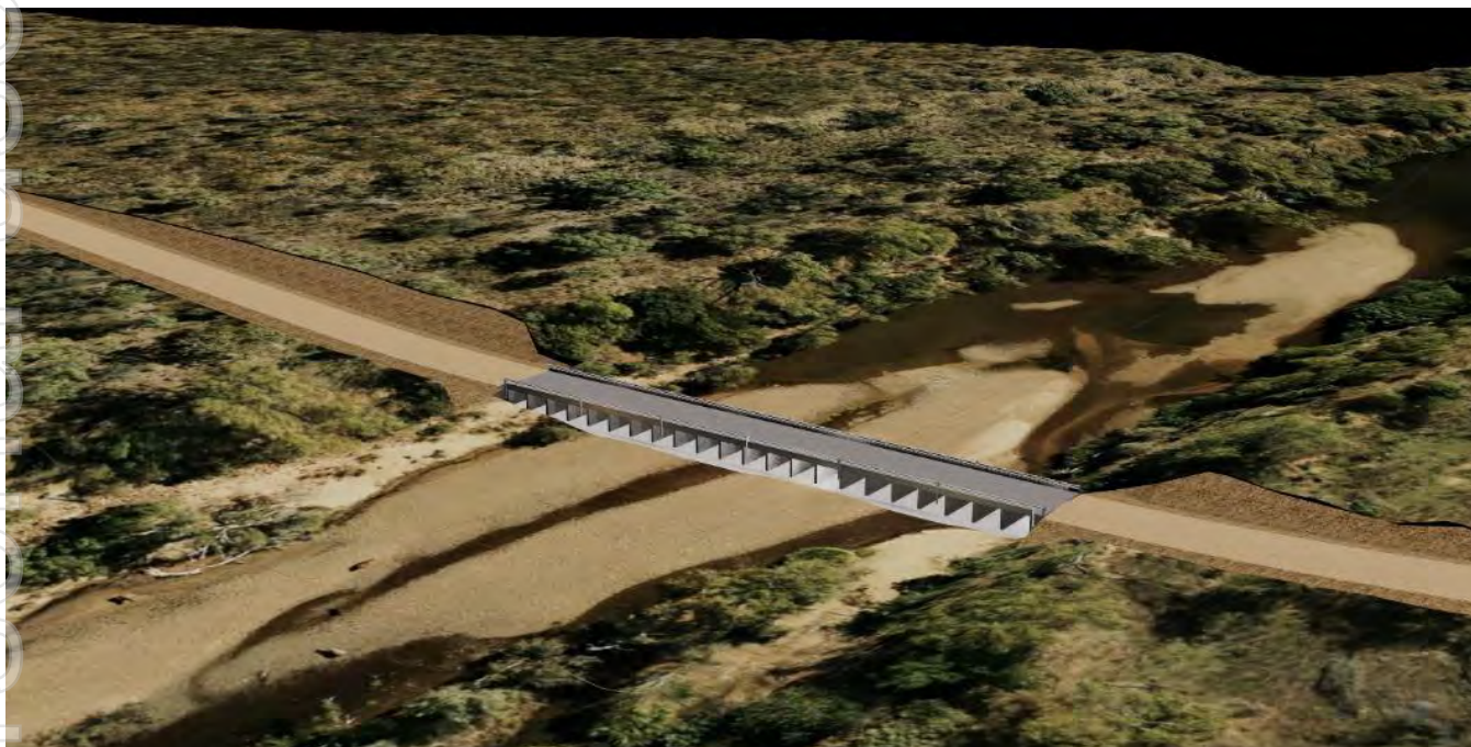
Figure 64: 3D model render of proposed Dunham River crossing, optimised to minimise impact on footprint, ecology and hydrology of the river.
