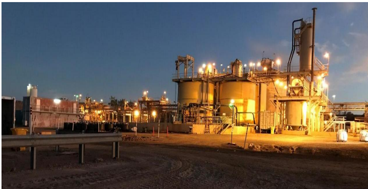
Figure A17: Existing CIL and Adsorption Tanks and Elution Column
