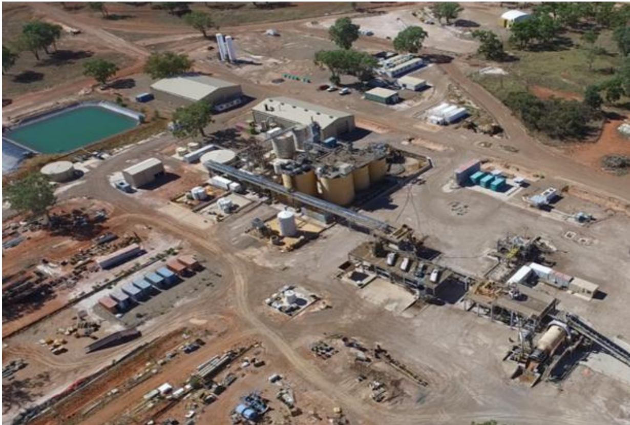
Figure 3: The existing Wonawinta Processing Plant.
