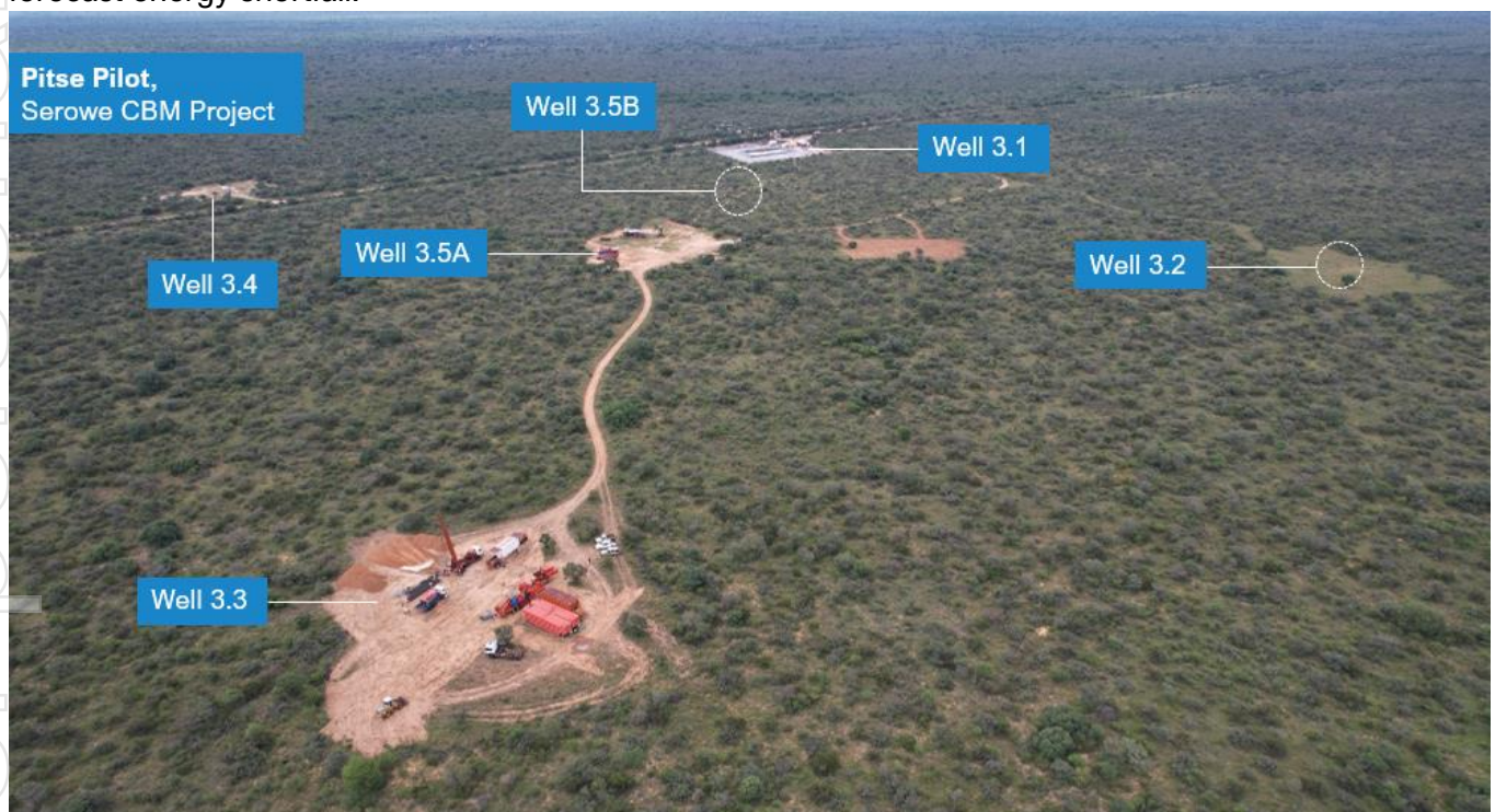
Figure 2. The Phase-1 Pitse Pilot at Botala's Serowe CBM Project in Botswana is a "proof-of-concept" to establish a production pathway to 3.5 petajoules of LNG per year. (Source: Botala)
