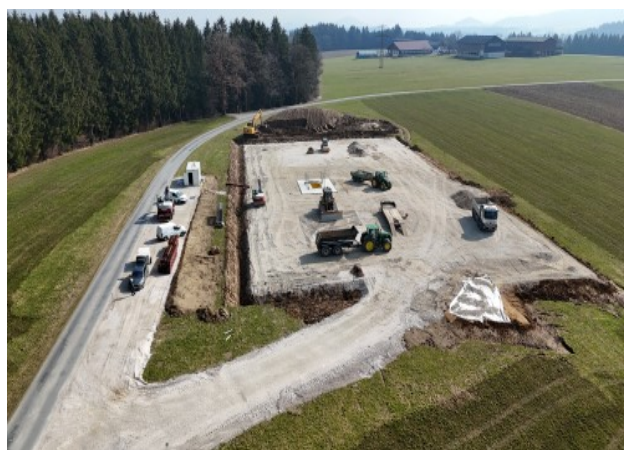
HOCH-1 rig site construction in the ADX-AT-I Licence during February 2026 in preparation for the commencement of drilling in April 2026
