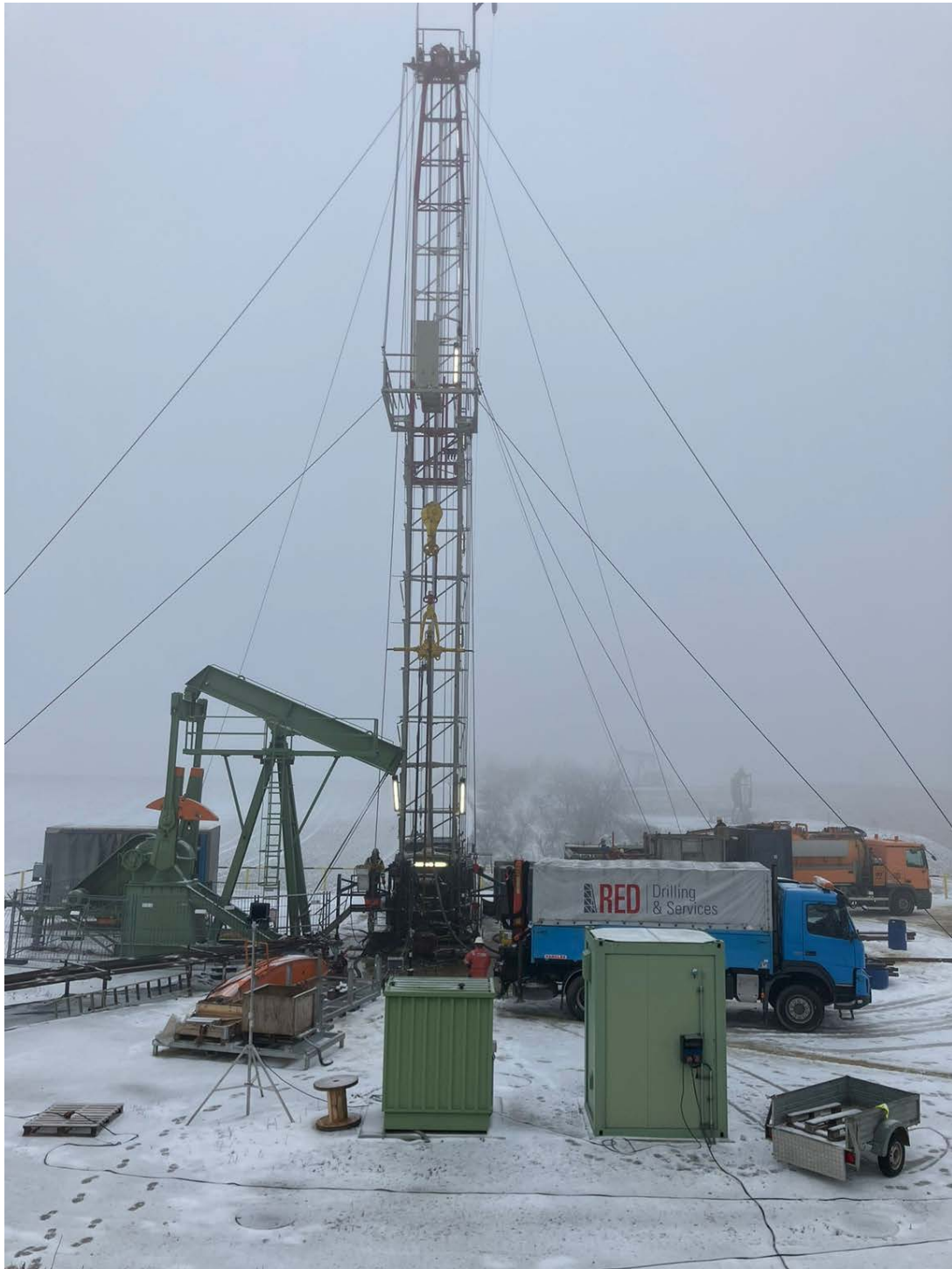
Figure 6: Work over operations at the Vienna Basin Oil Fields during December 2026
