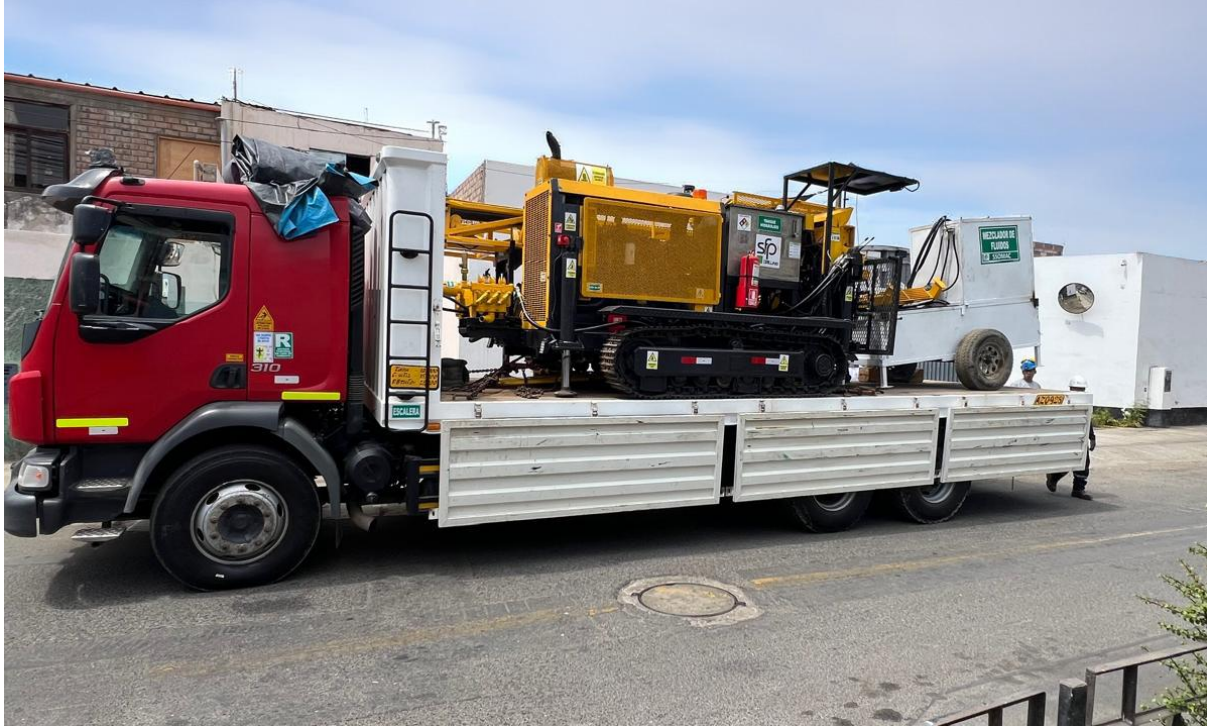
Photo 1. SFP Diamond Drilling Rig pre-mobilisation.
