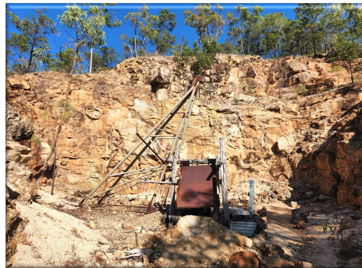
Daisy Bell open cut with exploratory shaft headframe still intact
