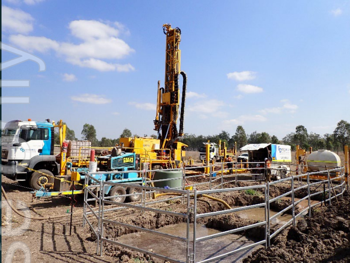
Active drilling campaign — Rolleston South, Nov 2025
