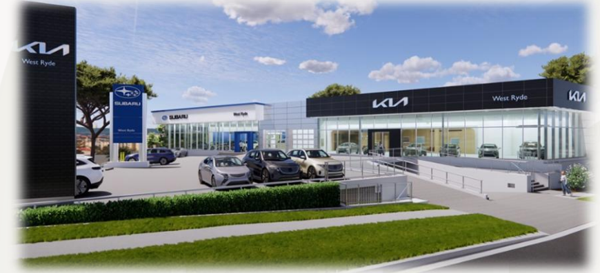
Ryde Kia & Ryde Subaru, Sydney – Under Construction
