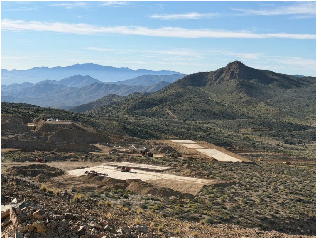
Figure 1: Equipment laydown area and other works at Colosseum
