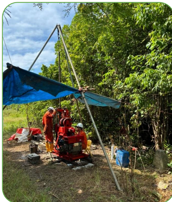
Figure 2: Soil Boring Test on access road
