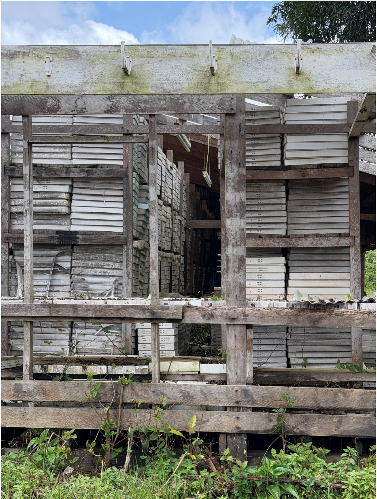
Figure 6: Close up of historic core shed from historic drilling at North Peters between 2005 – 2010 and core trays.
