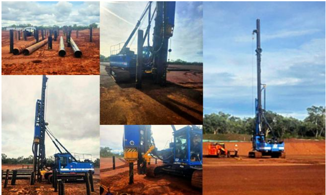
Piling to support the structural foundations of the gas plant
