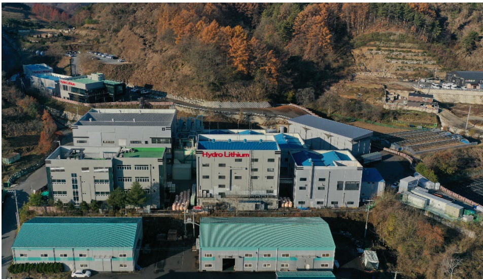
Figure 2: Hydro Lithium Refinery in Korea
