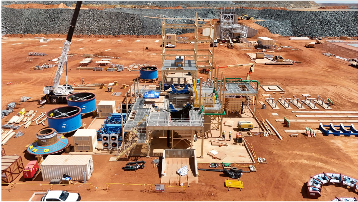
Mill and crusher areas with mill sections being placed.
