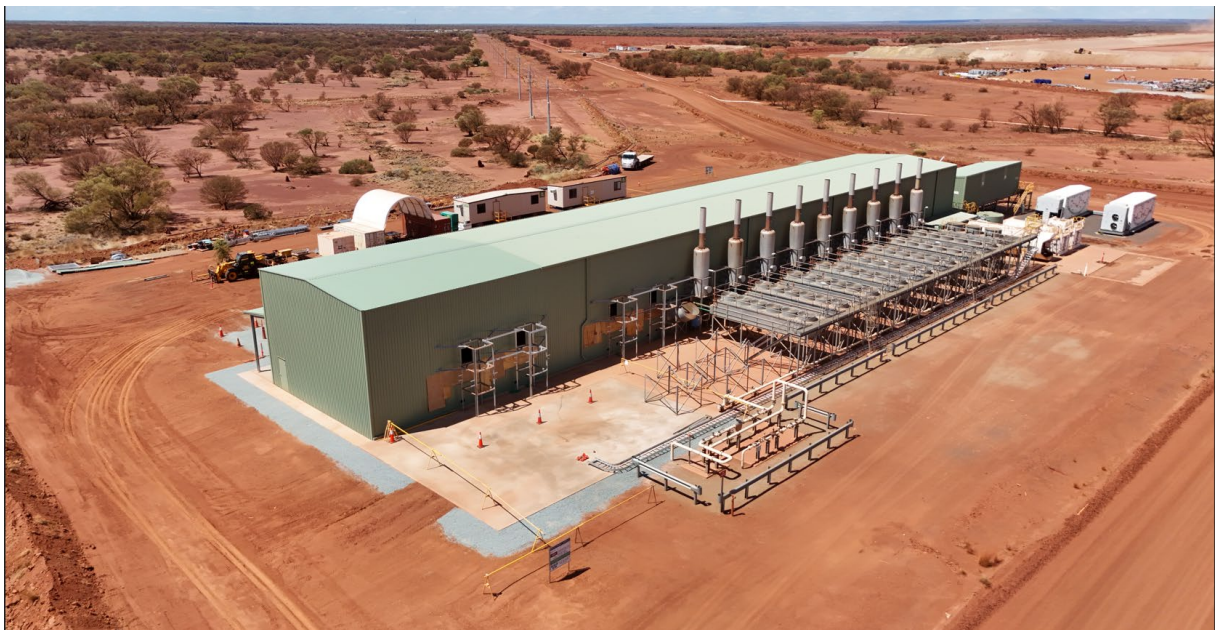
Power station extension.
