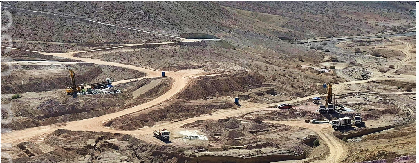
Two drill rigs in operation at the La Verde porphyry discovery, Cost Fuego copper-gold project, coastal Chile
