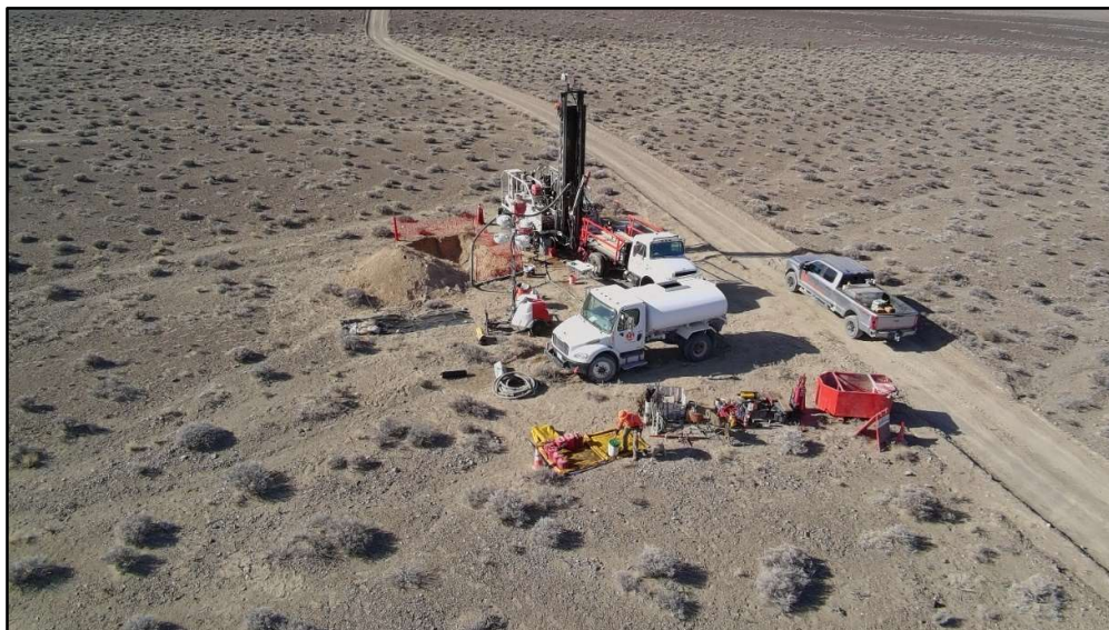
Figure 4. RC DRILL RIG ONSITE AT ALKALI FLATS
