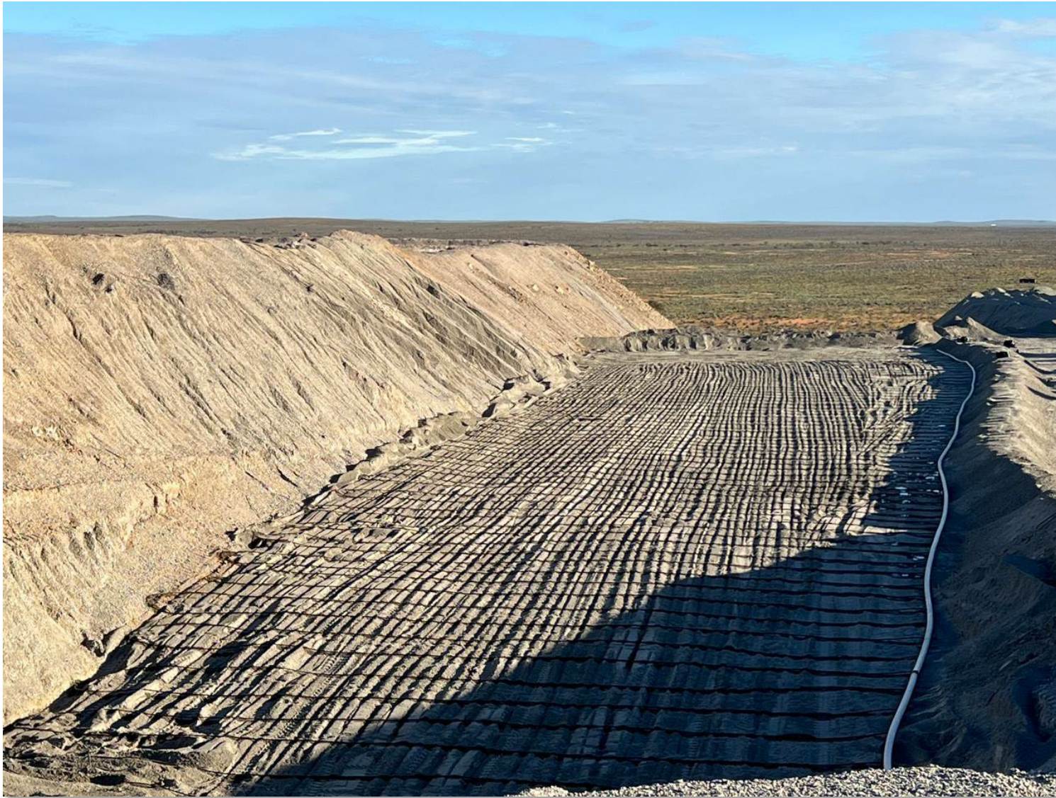
Photo 2: First re-crushed heap leach material now under irrigation
