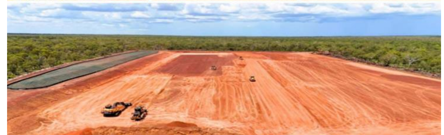
Early works for the Carpentaria Gas Plant including clearing, earthworks and refurbishment of equipment in Roma commenced in early October 2025
