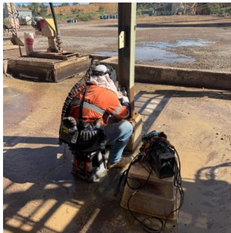
Figure 7: Steelwork repair across site
