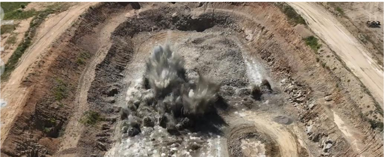
Figure 4: Blast BJS_317_02 at Blackjack South Pit on 8 th April 2026
