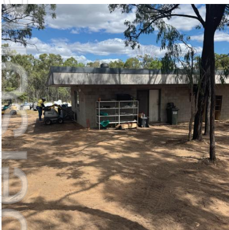
Figure 9: Caretaker House Converted to Geology Office
