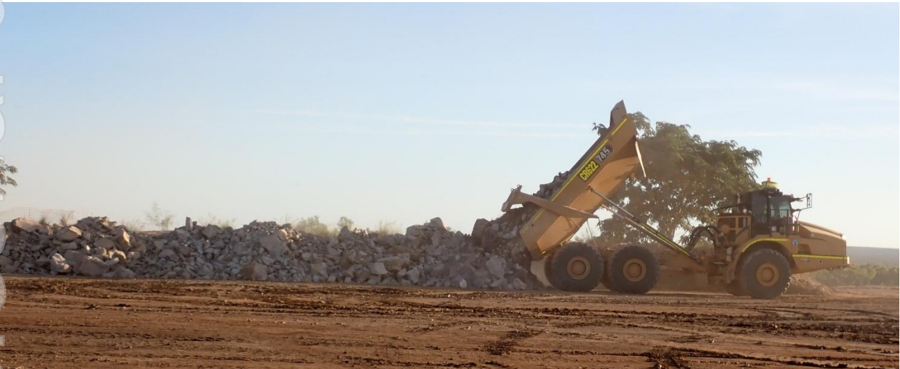
Figure 3: CAT745 offloading Blackjack south ore material to the ROM Pad (10 April 2026)
