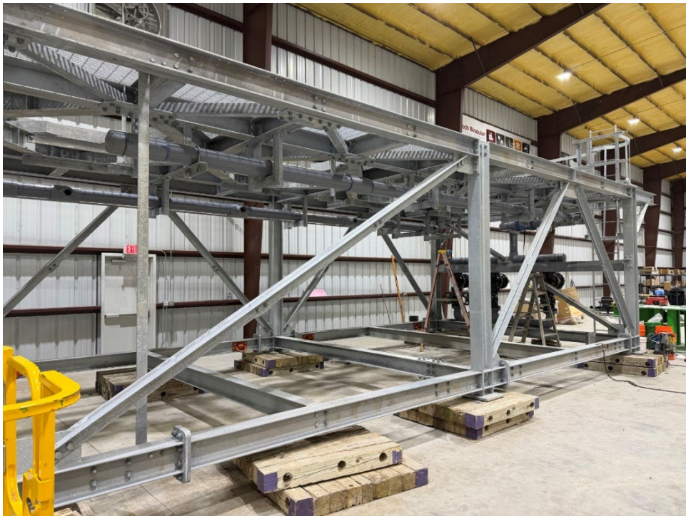
Figure 4: Construction of Li-Pro DLE Structure
