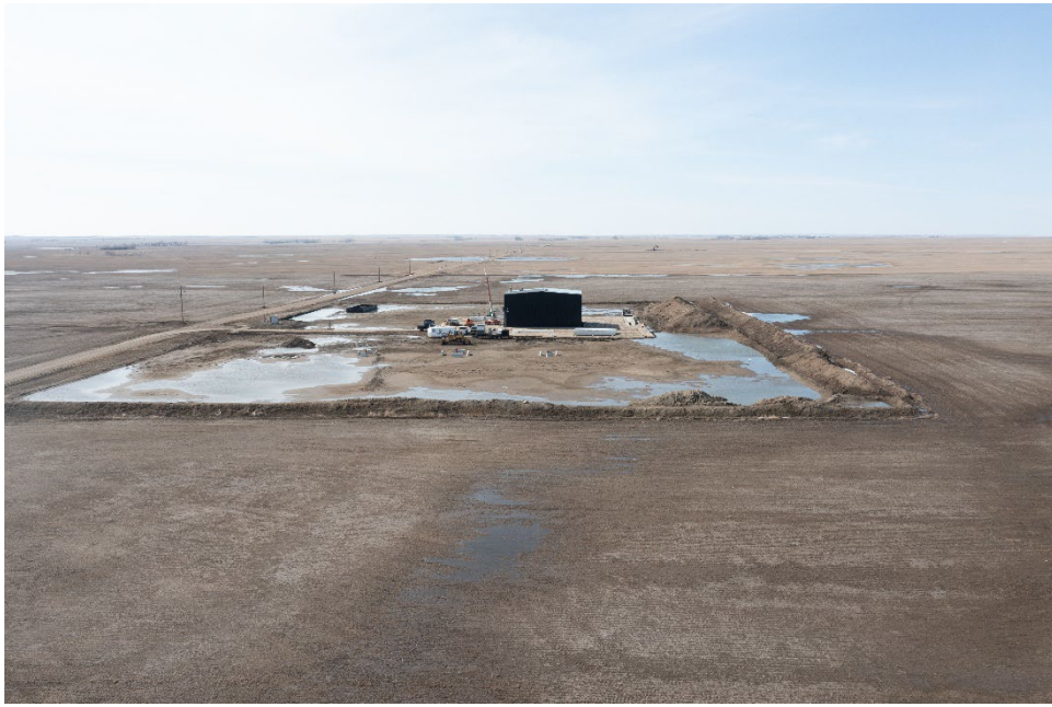
Figure 3: Aerial view of the facility during construction
