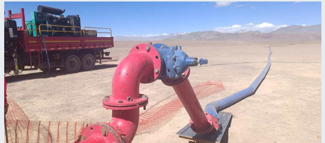
Water bore cleaning and pump testing at Nueva Esperanza, December 2025 - January 2026
