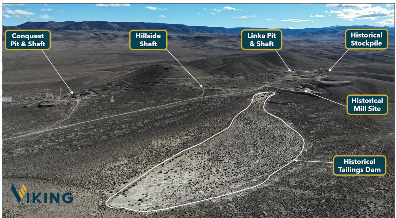
Figure 1; Photo of the Linka Tungsten Project showing historic mines, mill site, stockpiles and tailings dam.
