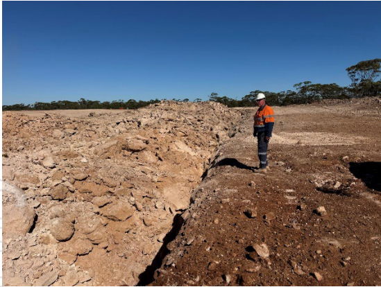
Inspection of blast area following blasting
