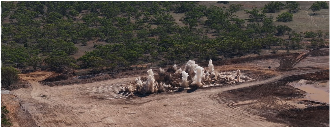
Controlled blasting taking place
