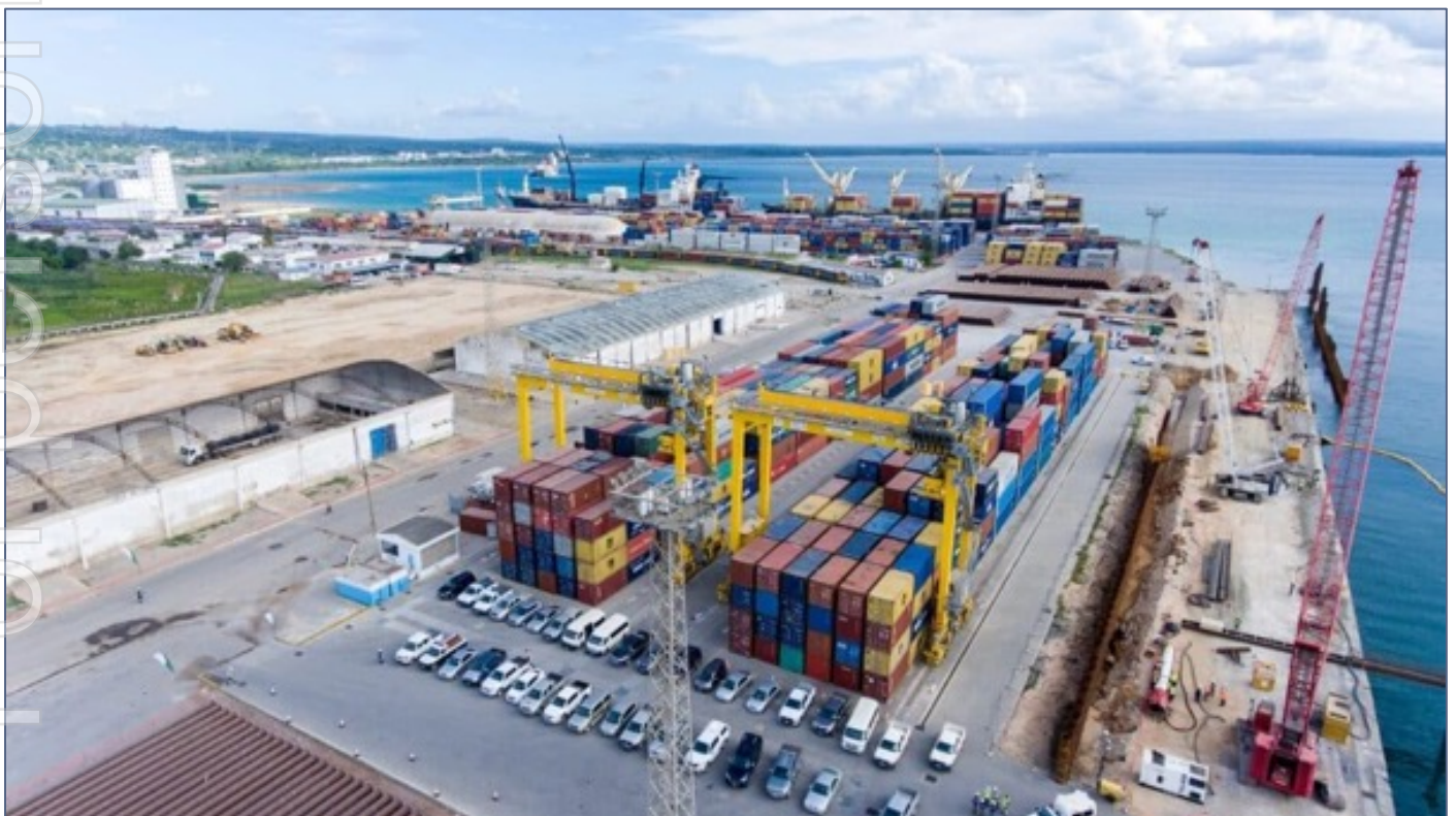
Figure 27: Port of Nacala, Mozambique
