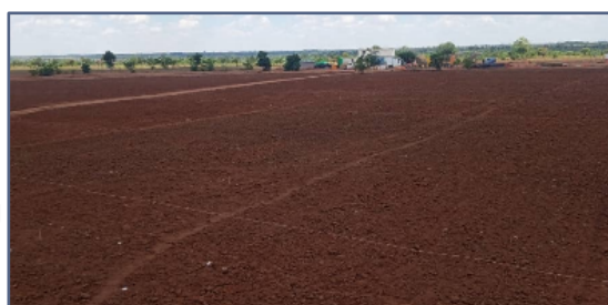
Test pit backfilling landforming
