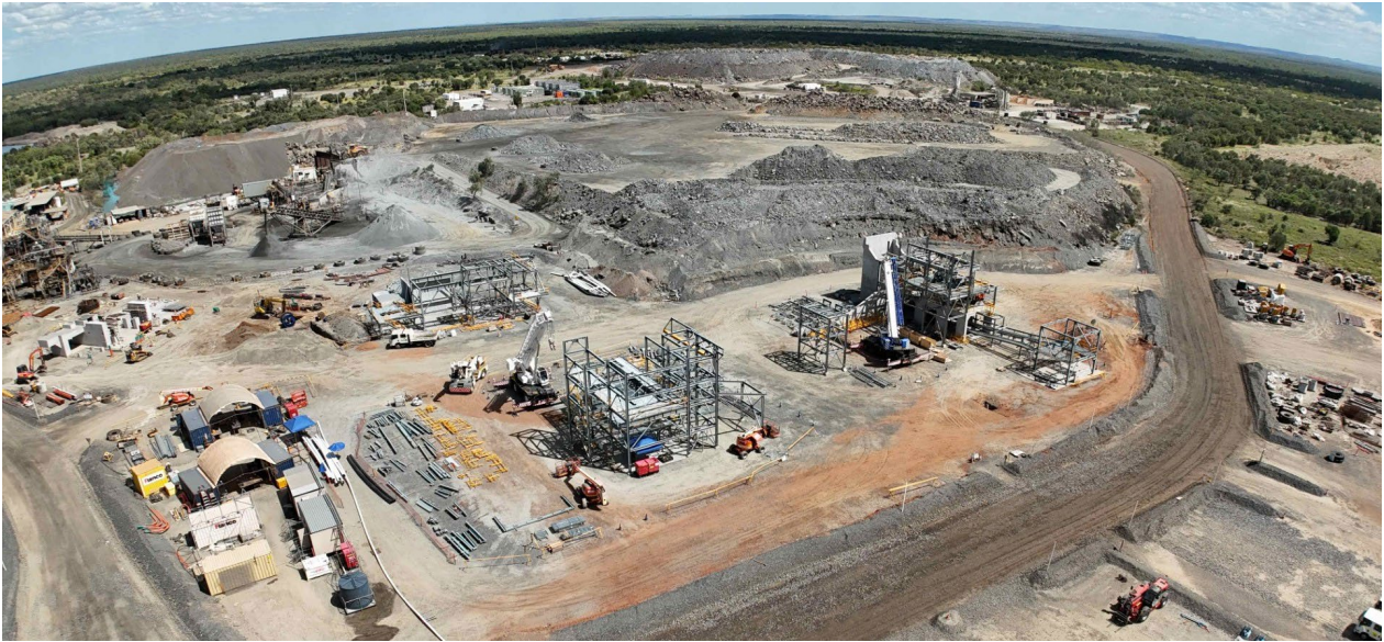
Photo 1: Current expansion work at Eloise. Ball mill raft concrete poured and backfilled (left), fine ore bin and emergency feeder (left-centre), screening and transfer area (front-centre) and primary crusher suspended slab concrete pour (right-centre).
