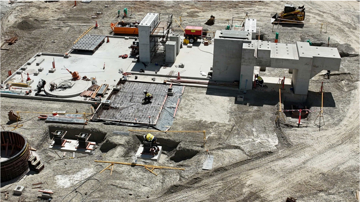
Photo 4: Ball mill area major concrete complete.
