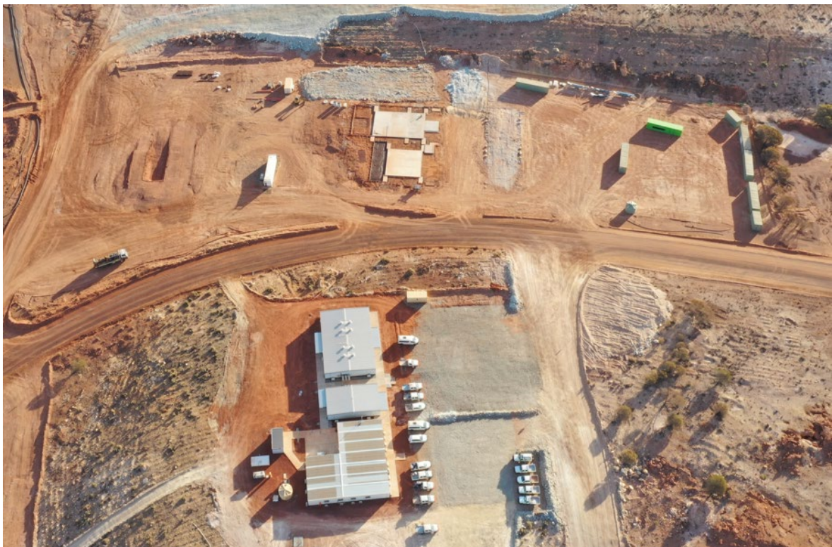
Figure 4 – Mining office and contractor workshops area advancing
