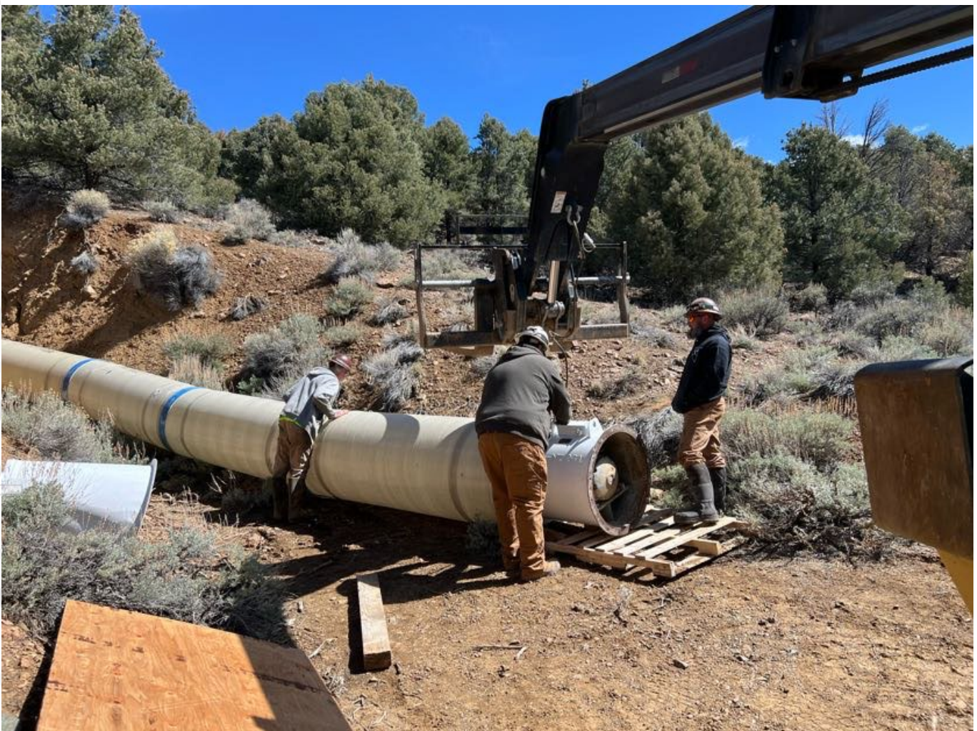
Photo 1 – Vent assembly and installation - Superior Level 4 Adit
