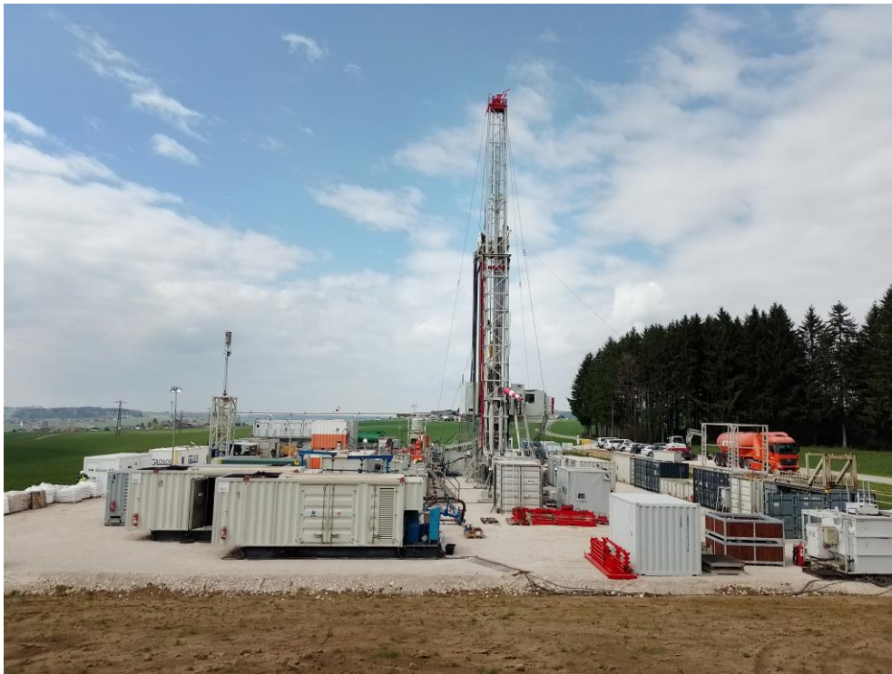
The MND Drilling & Services a.s. (MD-150) rig at the HOCH-1 drilling location prior to well spud
